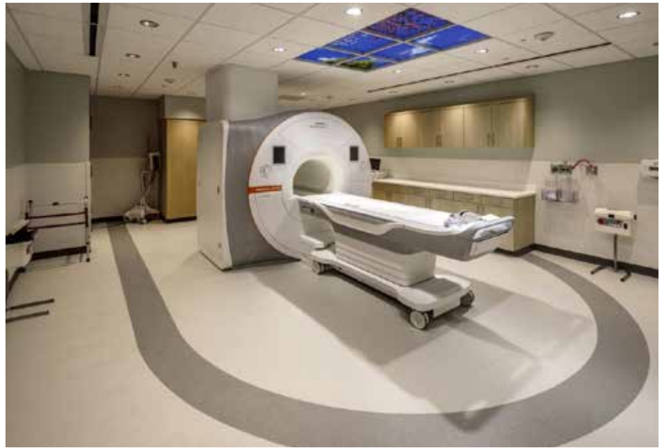
Corewell Health Pennock hospital's MRI room, the only hospital in Barry County (Adams 2025).
